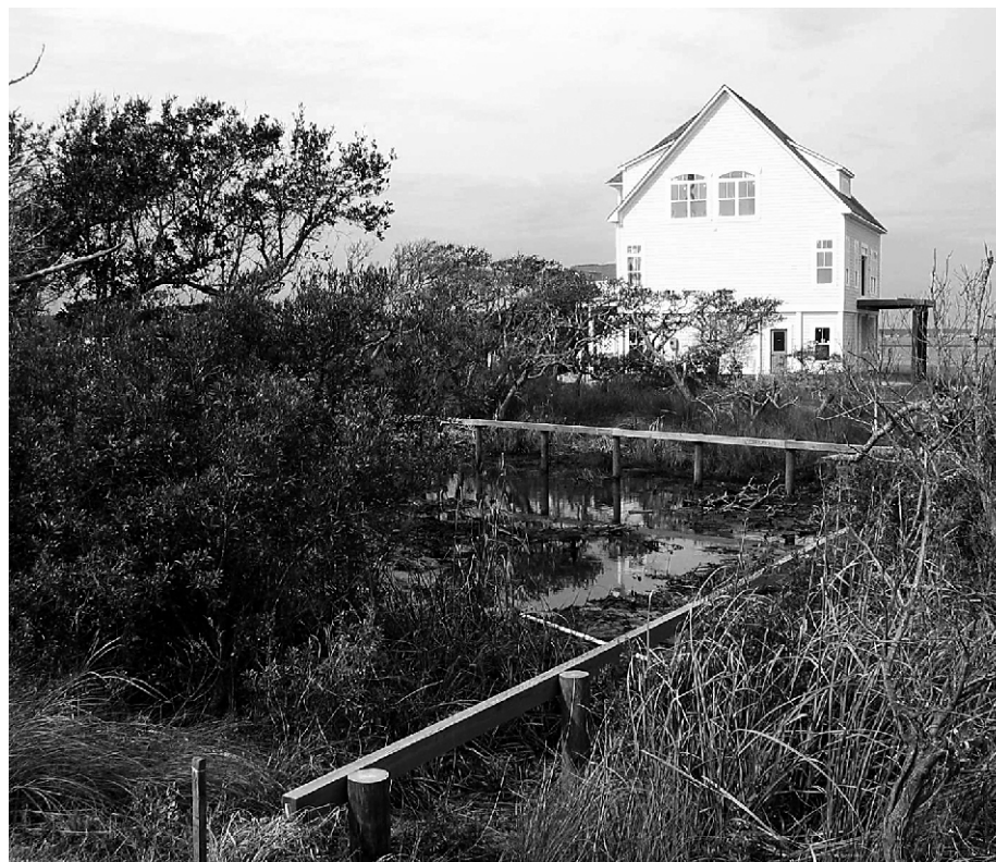
The state has forced the property owner to remove this bulkhead in Atlantic Beach.
