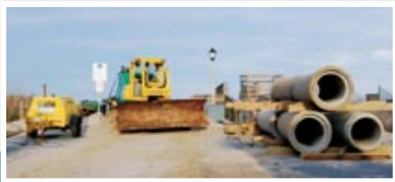
below: Runoff triggers a plume of pollutants in the ocean off the Outer Banks. left: N.C. DOT begins building a pipe to dump stormwater into the ocean.
