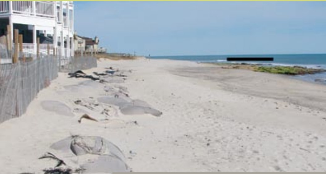
Twenty-year-old sandbags flank The Riggings condominiums in Wrightsville Beach.
