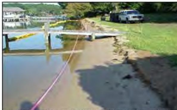
Bayou Texar, Pensacola FL prior to LS installation -2001
