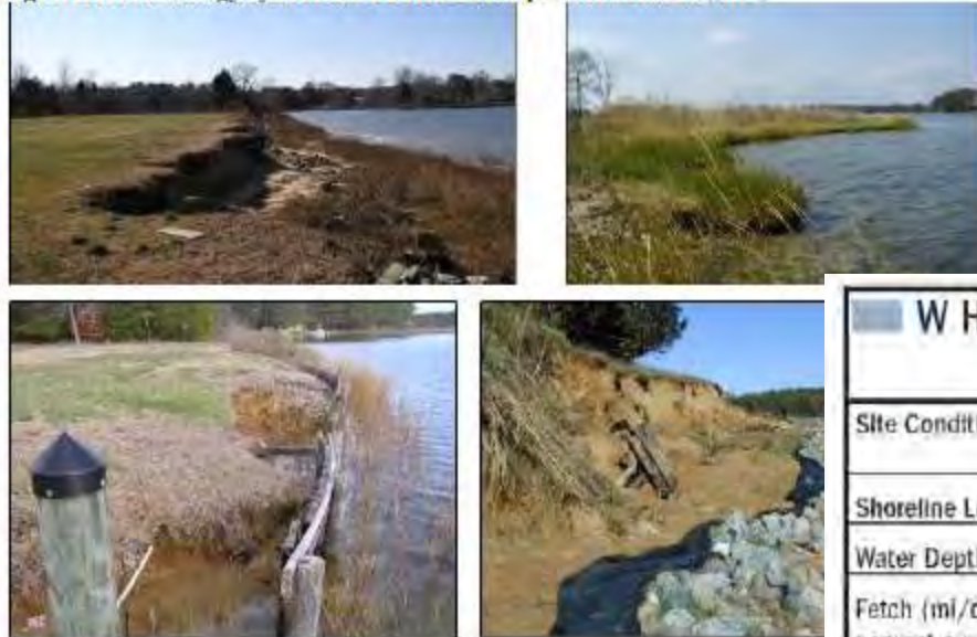
Figure 4: Low-energy systems and failed shore protection structures
